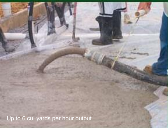
Hydraulic Squeeze Pump - Easy Clean Up
